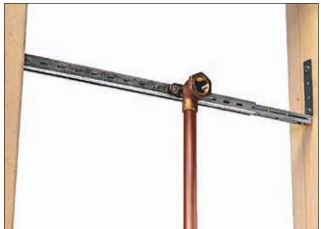
Figure 12-10 Shower Head Rough-In (Engineered)
