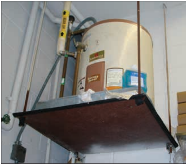
Figure 12-15 Makeshift Suspended Equipment Platform
