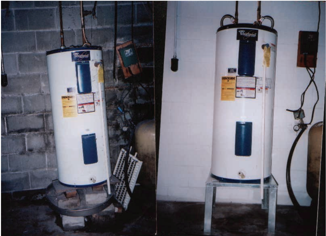
Figure 12-1 A Makeshift Attempt to Support a Water Heater versus an Engineered Solution
