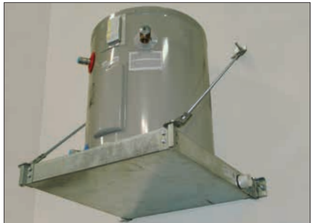
Figure 12-17 Engineered Wall-Hung Equipment Platform
