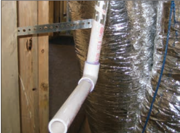
Figure 12-5 Condensate Drain Stub-Out (Poor)
