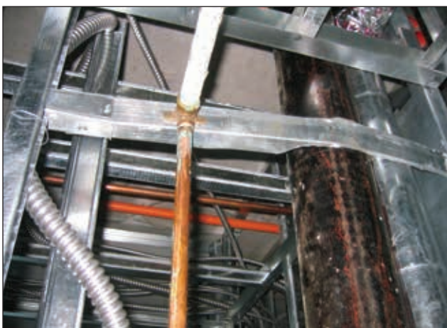
Figure 12-9 Shower Head Rough-In (Poor)
