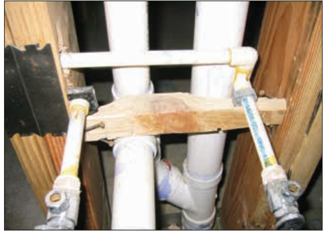
Figure 12-6 Sink Rough-In (Poor)
