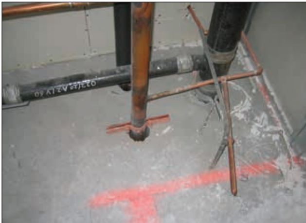
Figure 12-7 Toilet Rough-In (Poor)
