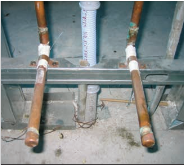
Figure 12-11 Poor Attempt at Dissimilar Metal Isolation
