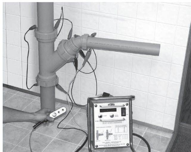
Figure 2-13 Fusion Lock Process in Operation
